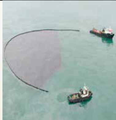
U-boom formation, note some oil is undercutting at the apex
